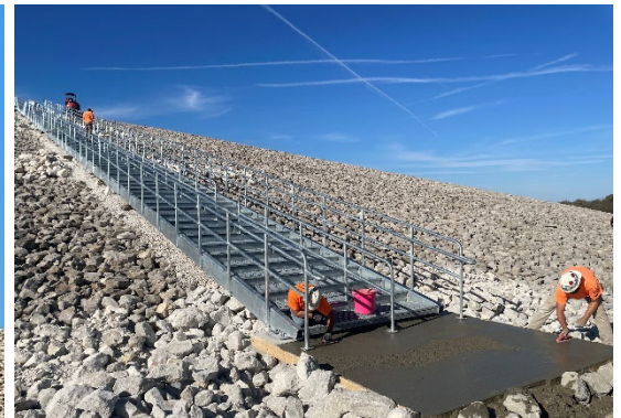
Finishing of concrete approaches
