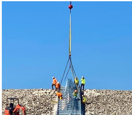
Placement of the final stair section using a 320 ton crane
